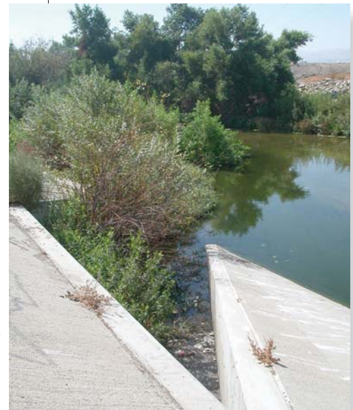
Stormwater runoff at storm drain
