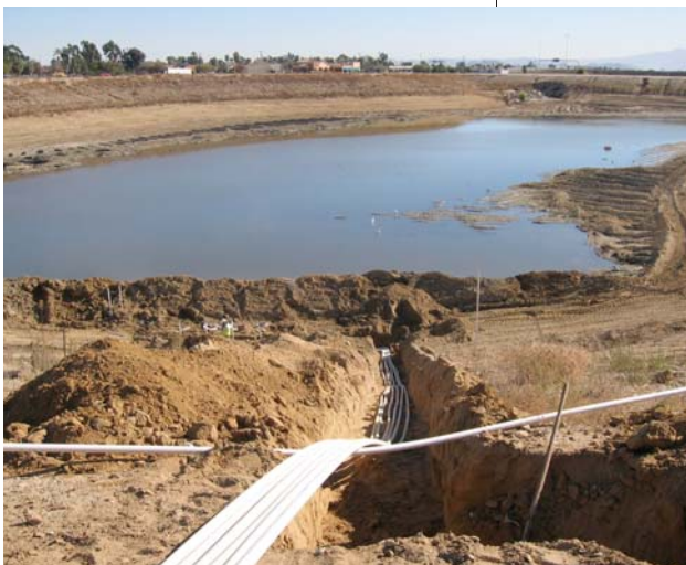
Lysimeters installation at Turner Recharge Basin
