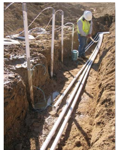
Lysimeter installation in Turner Basin
