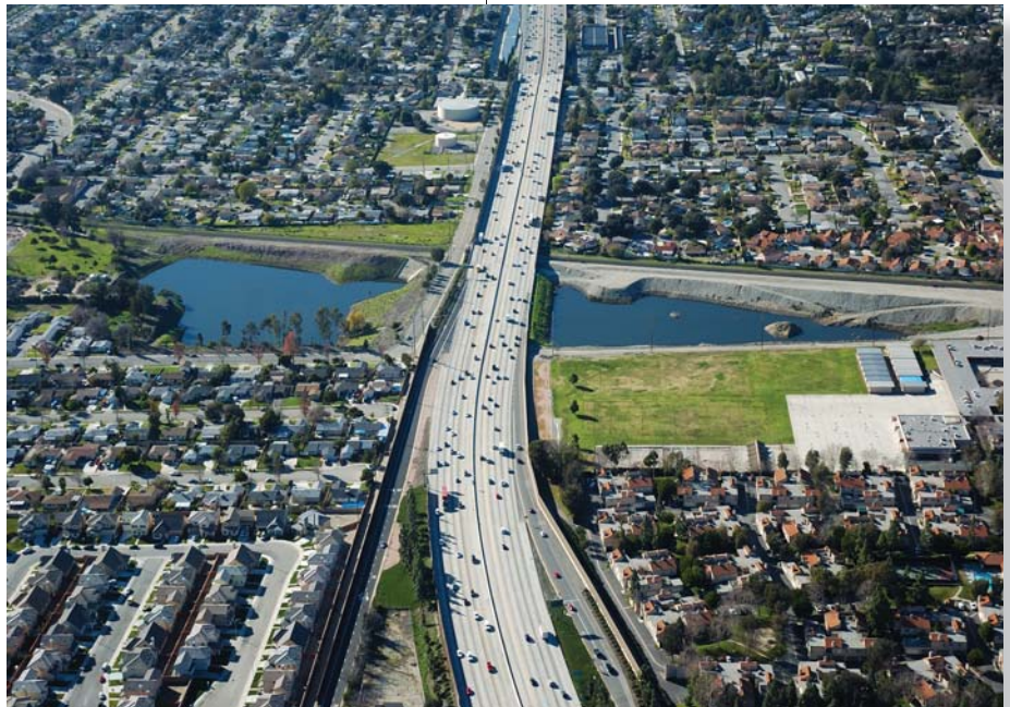
Artificial Recharge in the Chino Basin
