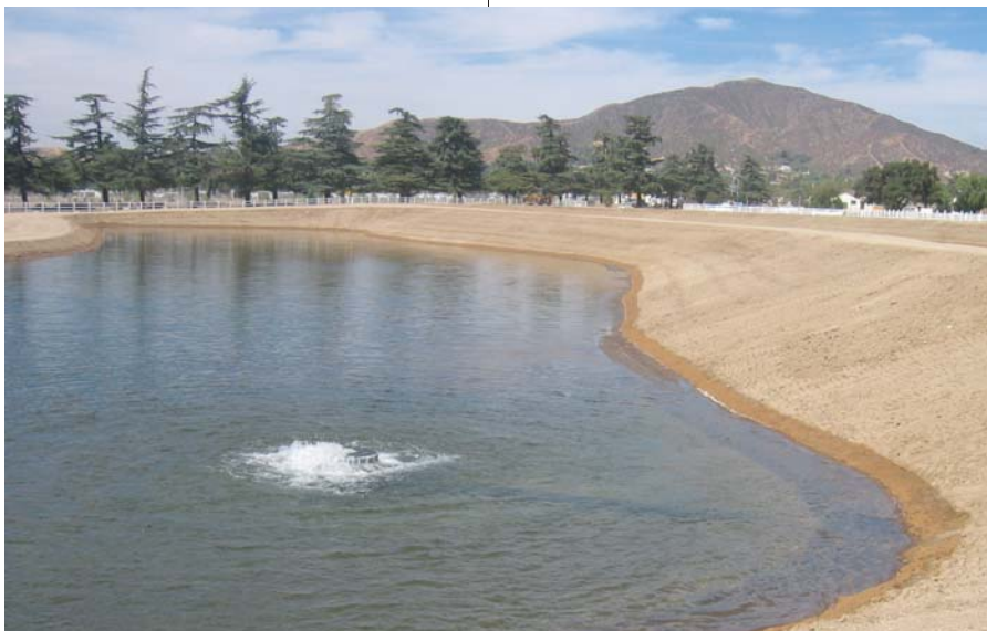
Recharge basin in the San Timoteo Watershed
