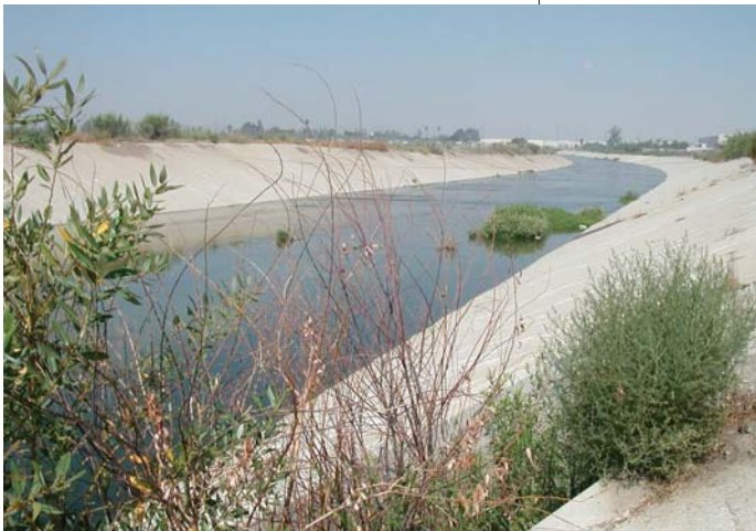
Stormwater runoff in channel
