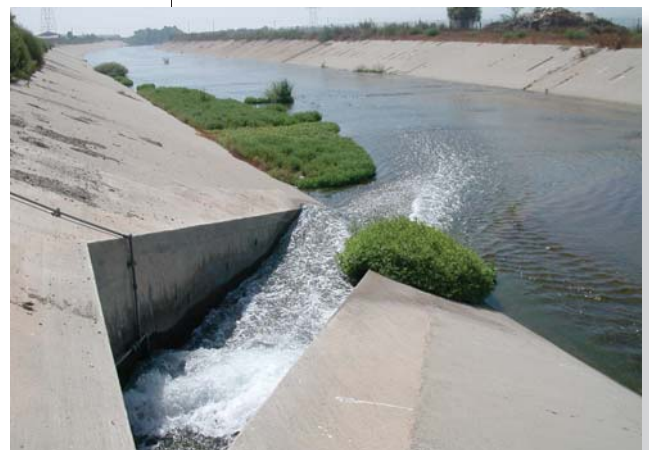
Chino Creek downstream outfall
