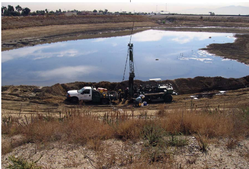
Lysimeters installation at recharge basin
