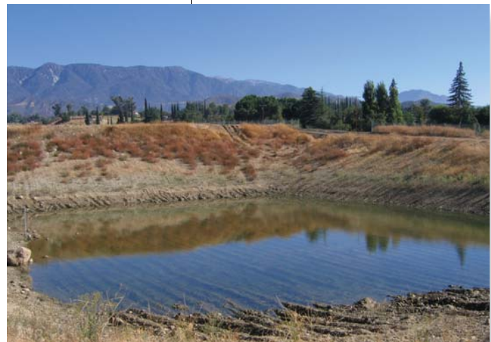
Recharge Basin in the San Timoteo Watershed
