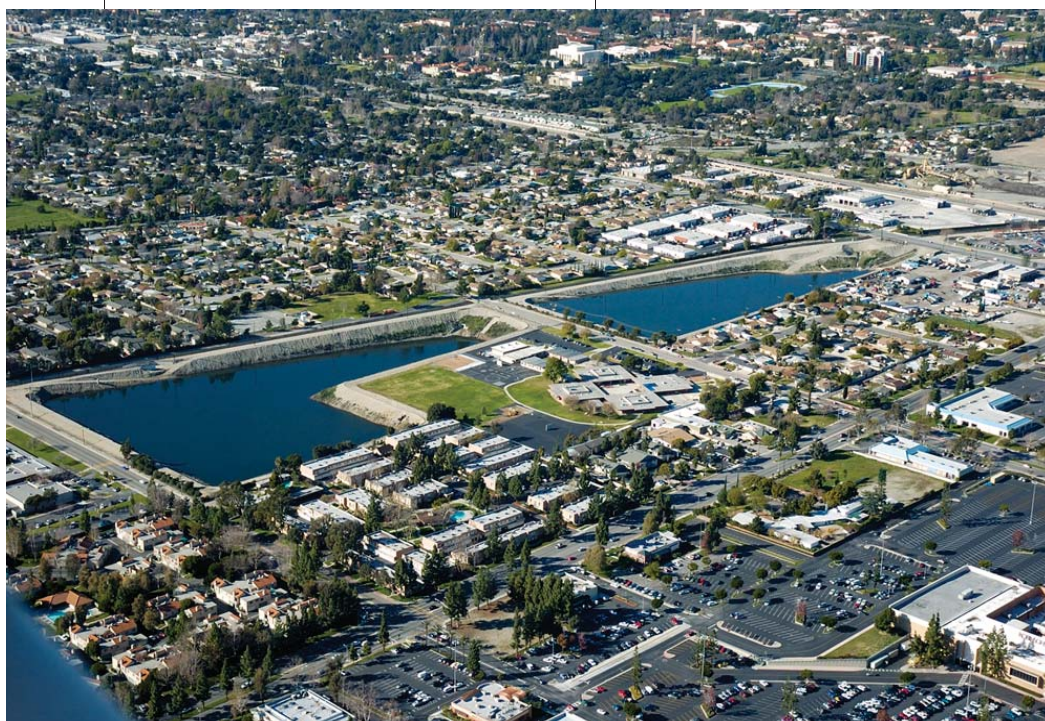
Artificial recharge in the Chino Basin
